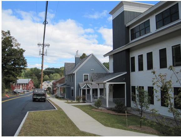
Algiers Village Affordable Housing- assessment and clean up led to twenty new units of affordable housing in Guilford; Photo Credit: Windham & Windsor Housing Trust
